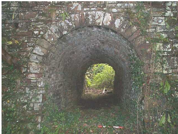
Shaft tunnel, part of a complex of mining remains at Pant y Geifr, Resolven.
